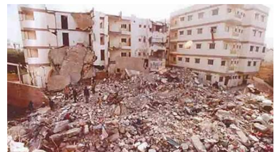
Bhuj earthquake- Gujrat, India, 2001 [33]
