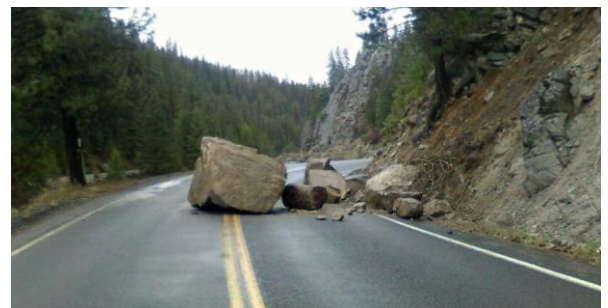
Rock slope failure [38]
